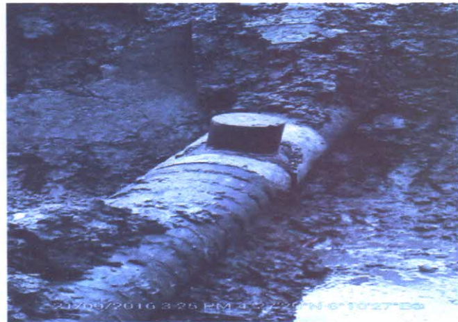
Figure 2: Coned after repair on the Pipeline .
