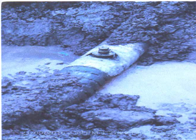
Figure 1: Cut-off cone on the pipeline.
